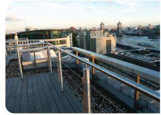
**ecodek**® were able to offer a solution to this in their Stadia profile. This solved the issue whilst enabling a continuation of matching material for the internal and external spaces.
